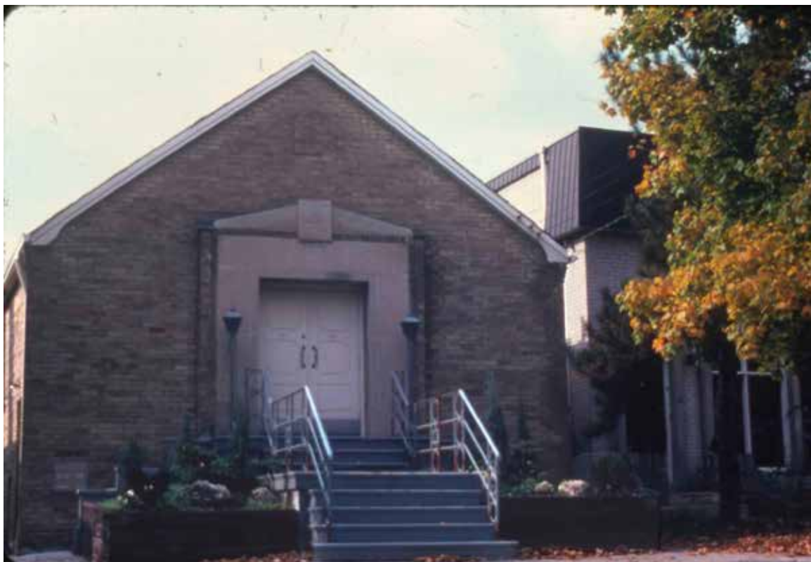
PRE-RENOVATION Exterior of 22 Gilgorn in the 1980s
